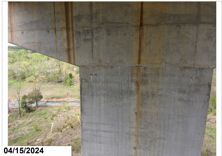
Bent 2, Back, Top of Pier Wall: cracking with efflorescence.
