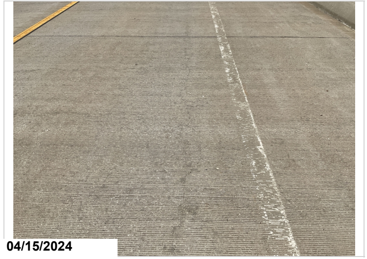
Spans 6 & 7: longitudinal cracking. CS2.
