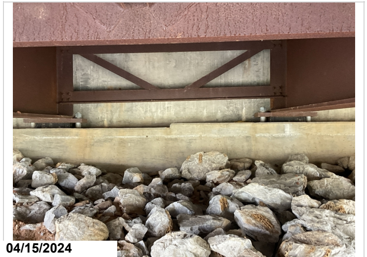
Abutment 1: Efflorescent cracking. CS2
