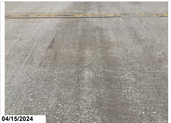
Span 5: transverse cracking. CS2.
