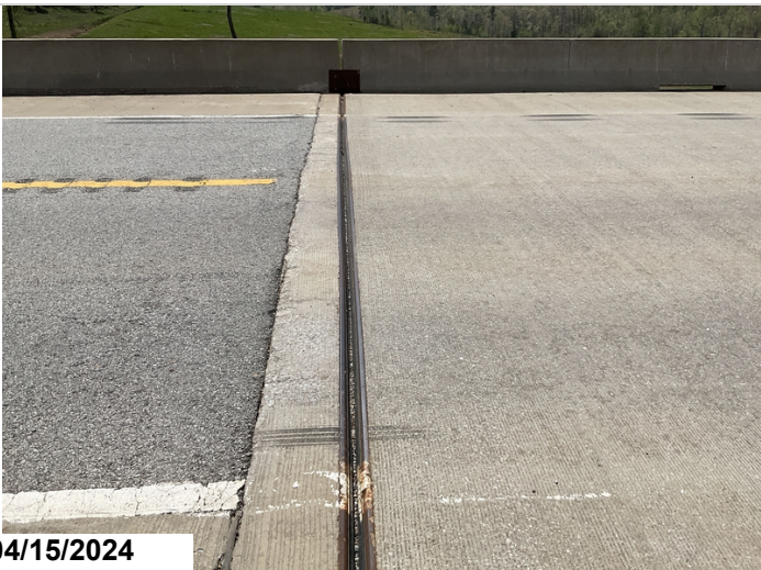
Joint at Abutment 1: Debris impactation. CS2.
