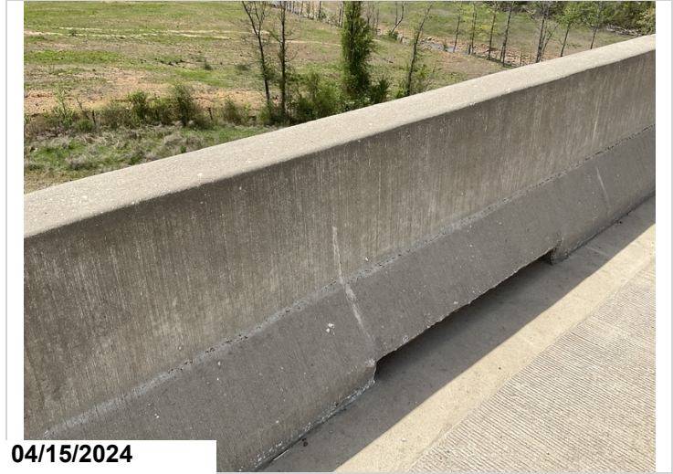
Bridge Railing: typical cracking with efflorescence. CS2.
