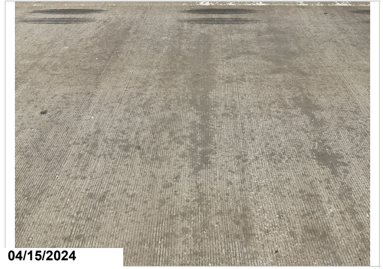
Span 3: transverse cracking. CS2.
