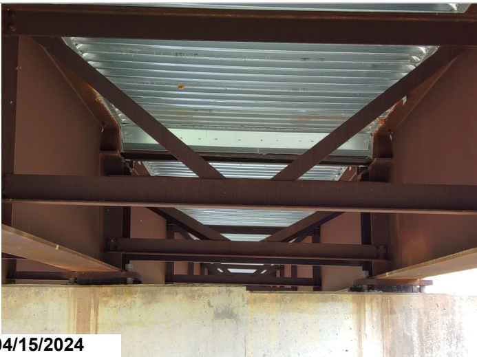
Typical Elastomeric Bearing.
