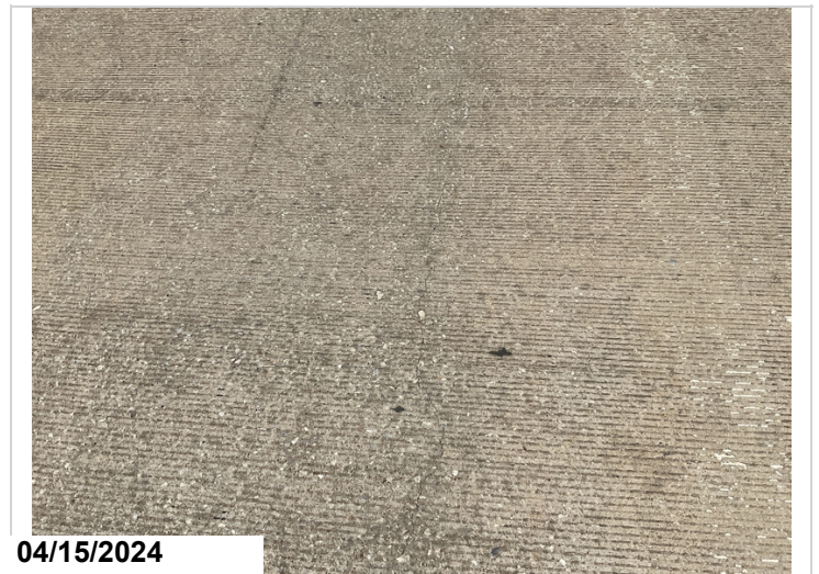
Span 2: longitudinal cracking. CS2.
