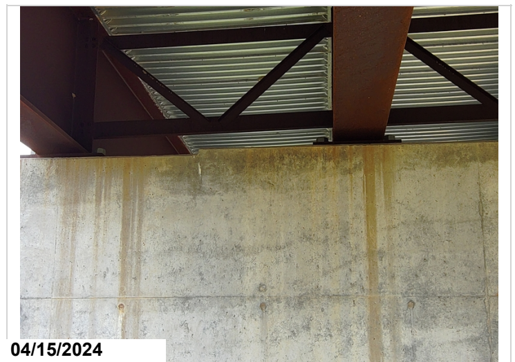
Bent 3, Pier Cap, Back: cracking with efflorescence. CS2.
