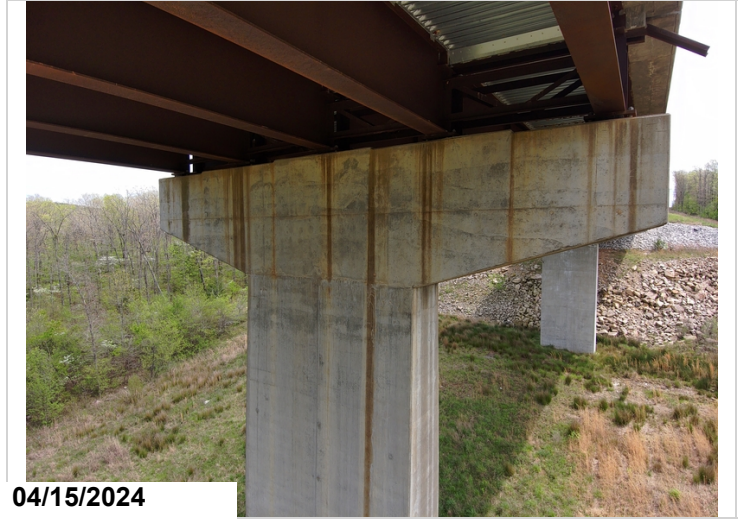
Bents 2 & 5: rust staining on Pier Cap from Assembly Joints without Seals.
