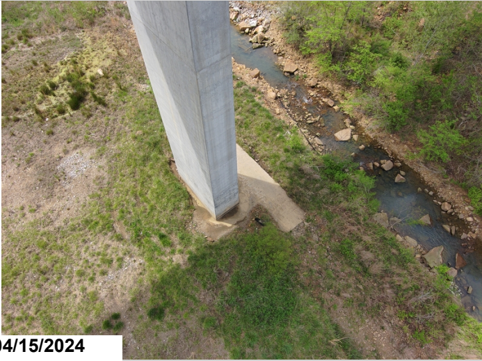
Bent 3: exposed Footing.
