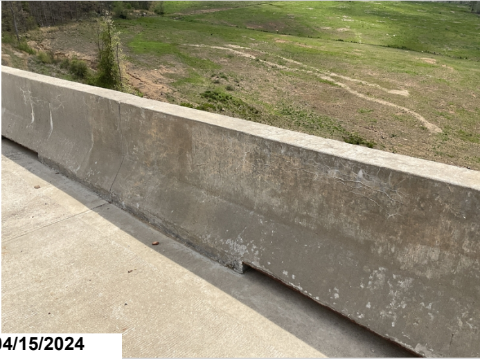
Span 3, Left Bridge Railing: map cracking with efflorescence. CS3.
