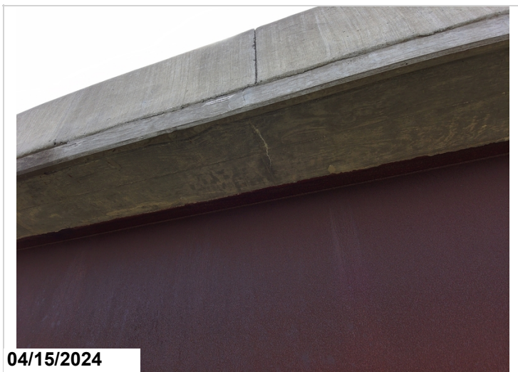
Deck, Right & Left Overhangs: cracking with efflorescence typical throughout the structure. CS2.
