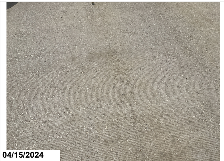
Span 3: longitudinal cracking. CS2.
